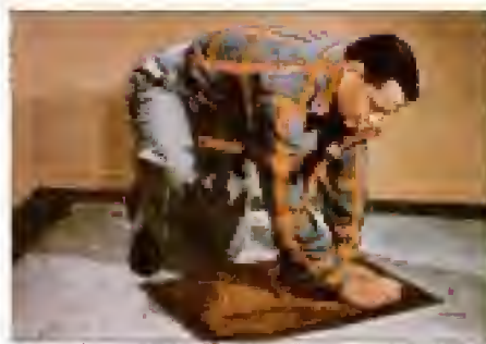
2. Mark the Formica sheet to size for the new top.
